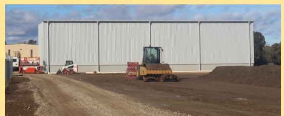
New Faucet Stroman shed in Tate Drive, Kerang
